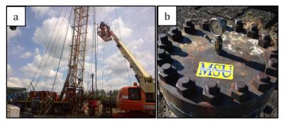
**Figure 1. a)** Filling the bailer with ureolytic microorganisms for delivery downhole. **b)** 9 5/8" Gorgas #1 well head.
